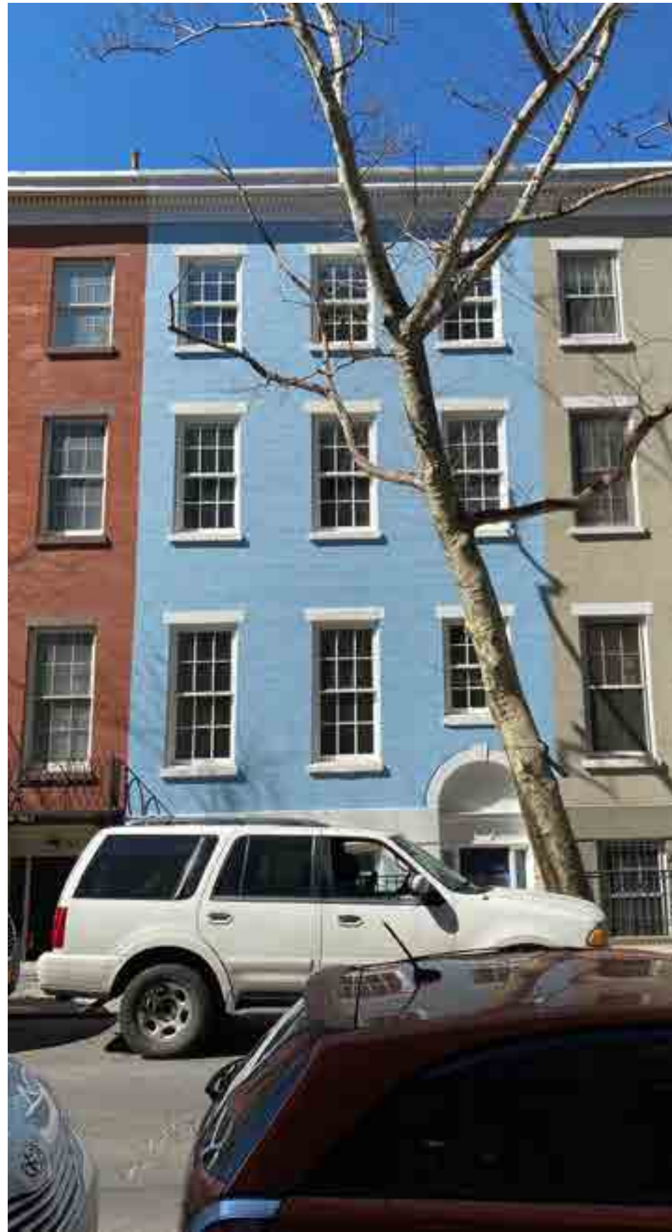
186 Sullivan Street Facade
