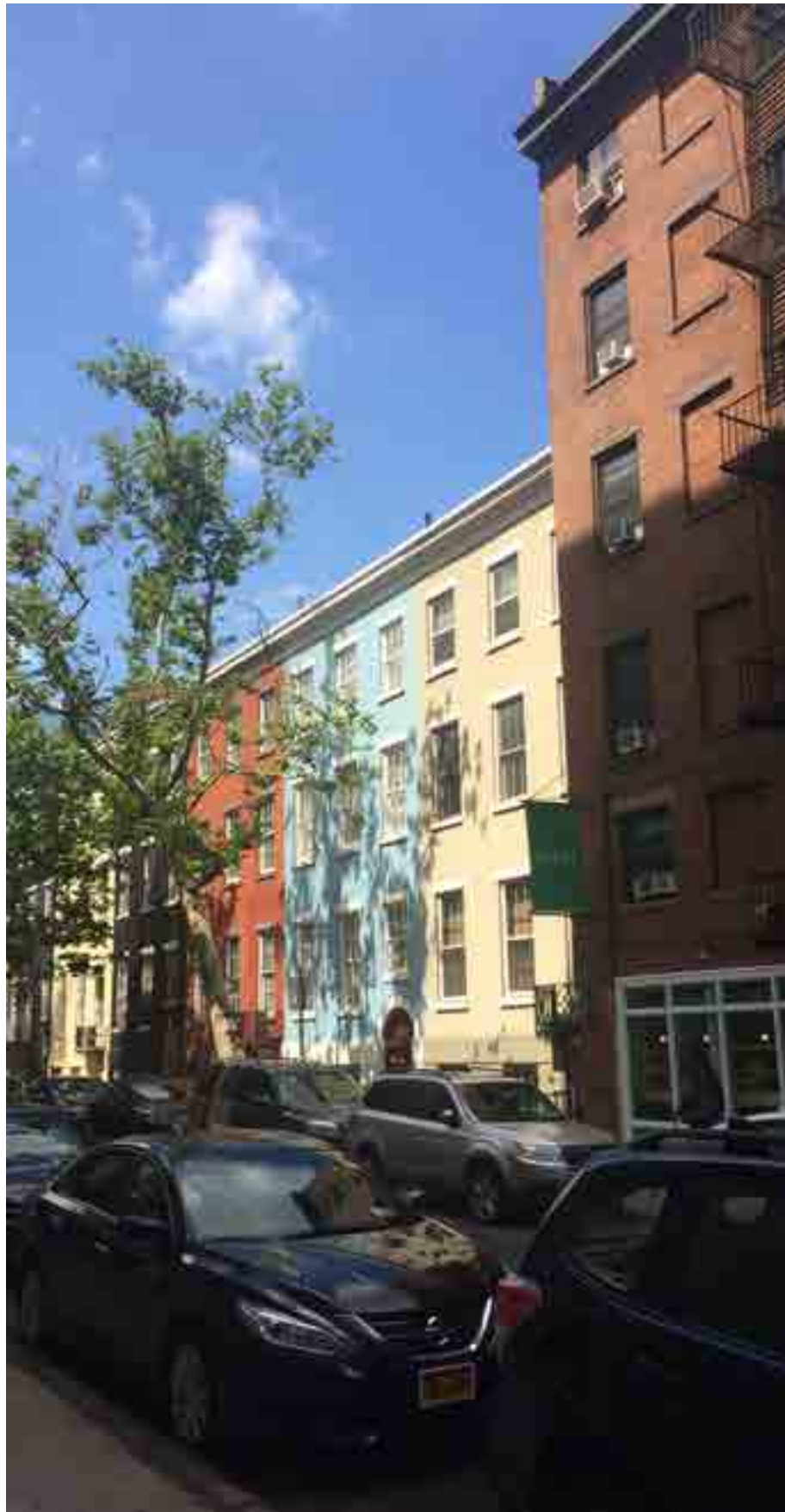
Sullivan Street Facing Southwest
