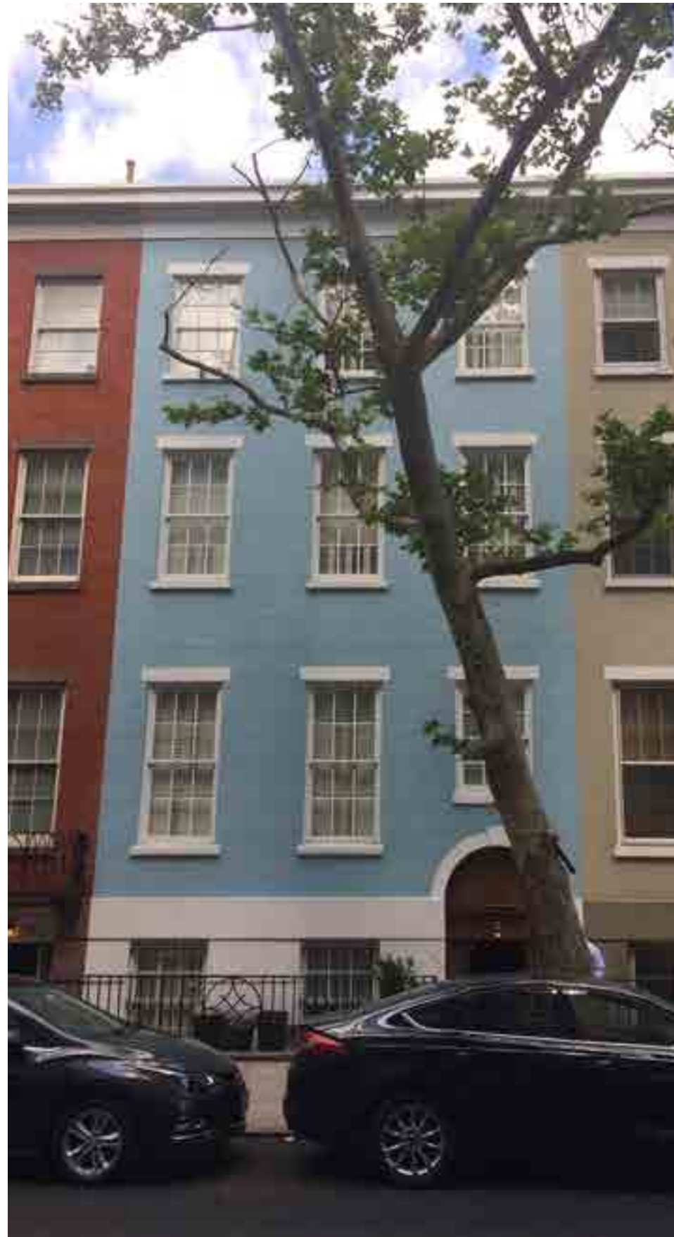
186 Sullivan Street Facade
